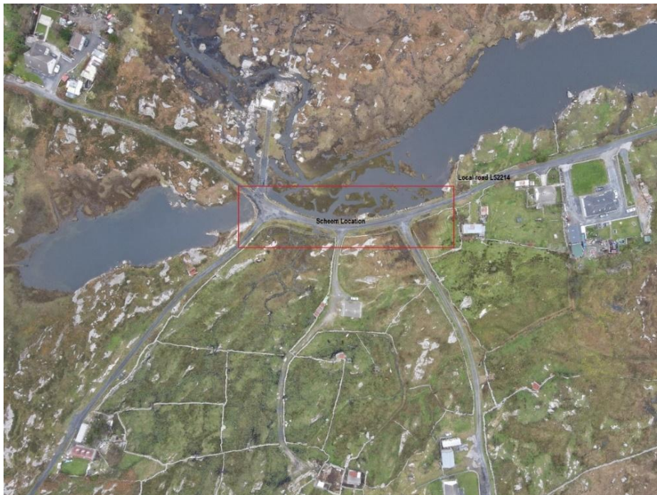
Figure 2.2 Aerial view. March 2025
